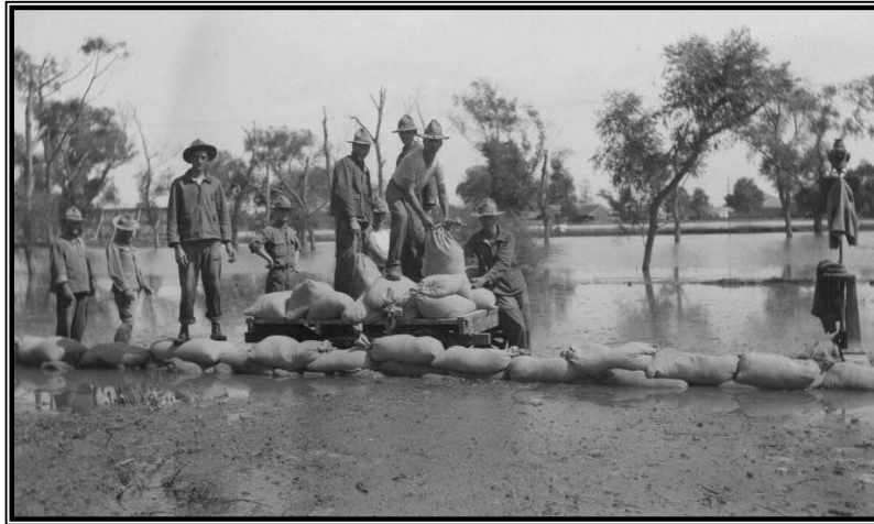
Figure 2 – Soldiers doing repairs to the levees after the 1916 flood near Brownsville
